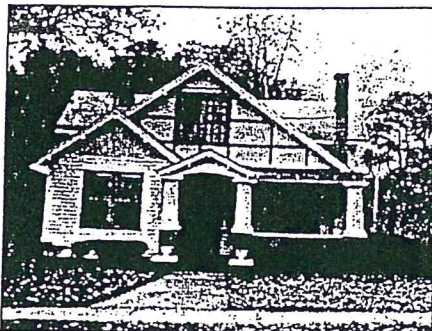
Craftsman style: wide eave overhang with rafter tails often exposed, decorative (false) braces are common under gables, tapered, square columns are common.
